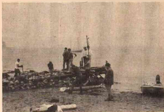
Groundwork, well under way, for construction of our docking facilities on Frog Island. This job took an entire day, using rocks and driftwood.
